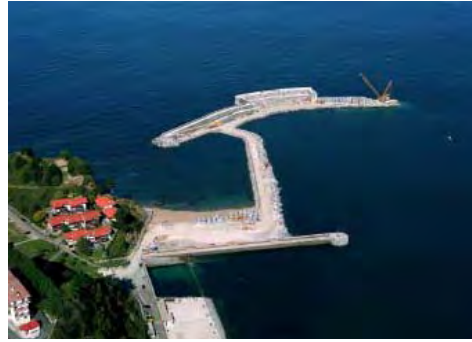
Figure 7-27: Mutriku OWC Breakwater – Bilbao, Spain
